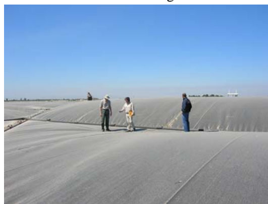
Picture below: the 7 acre digester cover
