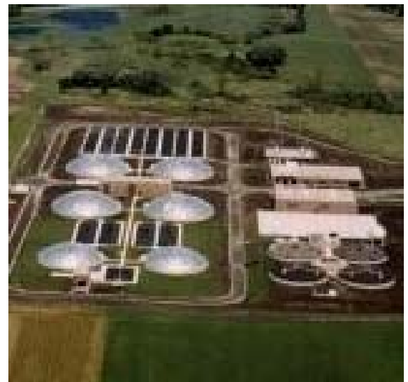
Albert Lea Wastewater Treatment Center Albert Lea, Minnesota
