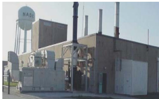
NADC Cogeneration Facility
