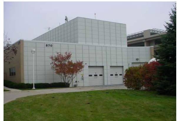
Centralized Building Plant
