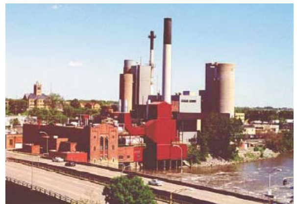
University of Iowa Cogeneration Plant
