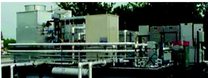
(Left) Early test of small cogeneration featuring a microturbine and absorption chiller on the roof of an Indianapolis drugstore. (Right) Fuel cell in Central Park in New York.
