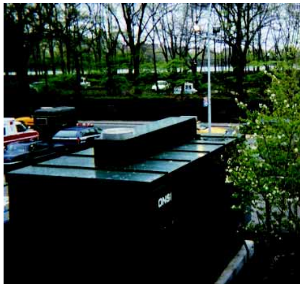
(Left) Early test of small cogeneration featuring a microturbine and absorption chiller on the roof of an Indianapolis drugstore. (Right) Fuel cell in Central Park in New York.
