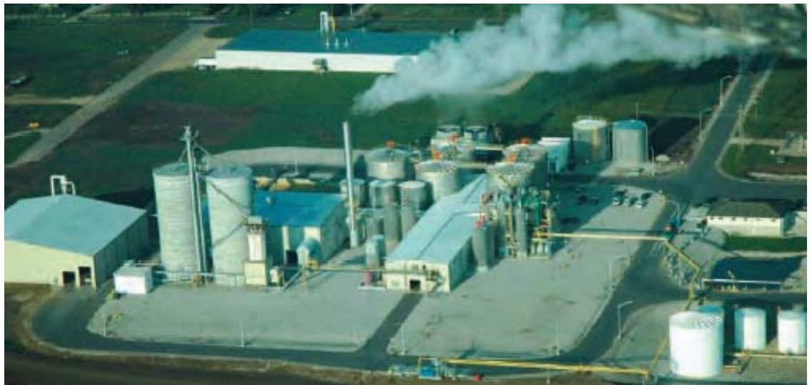
East Kansas Agri-Energy (EKAE) Ethanol Plant – Garnett, Kansas
