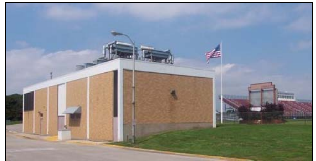
Maine South High School CHP Facility
