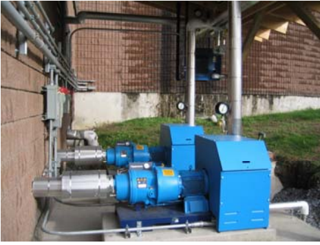
Dual alternating CompAir V07G compressors
