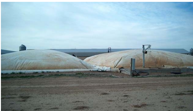
The anaerobic digester at Colorado Pork
