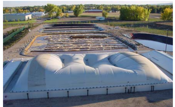
New Belgium Brewery's 80,000 gallons/day process water treatment plant with anaerobic and aerobic digestion
