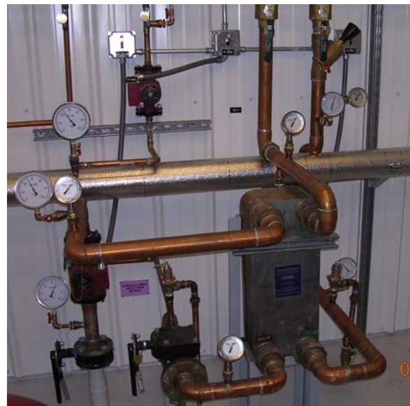
Figure 3: Heat Recovery System
