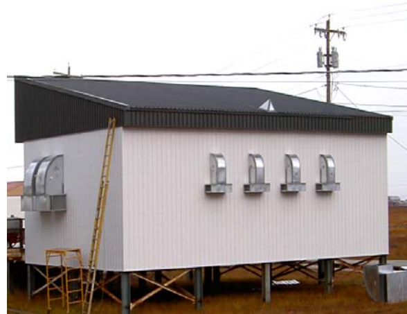
Figure 1: Kwigillingok Power Plant
