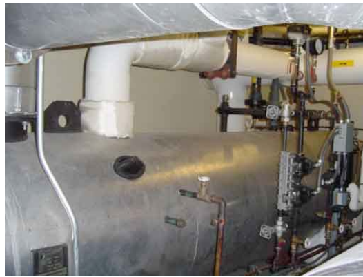
Heat Recovery Steam Generator
