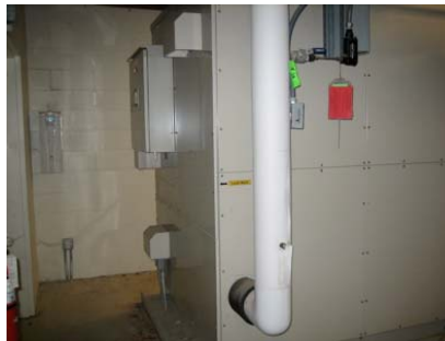
Nishiyodo adsorption chiller
